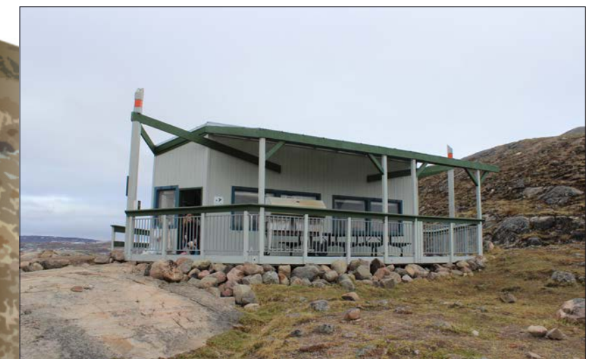
PAVILION EXISTING CONDITION - JUNE 2019
